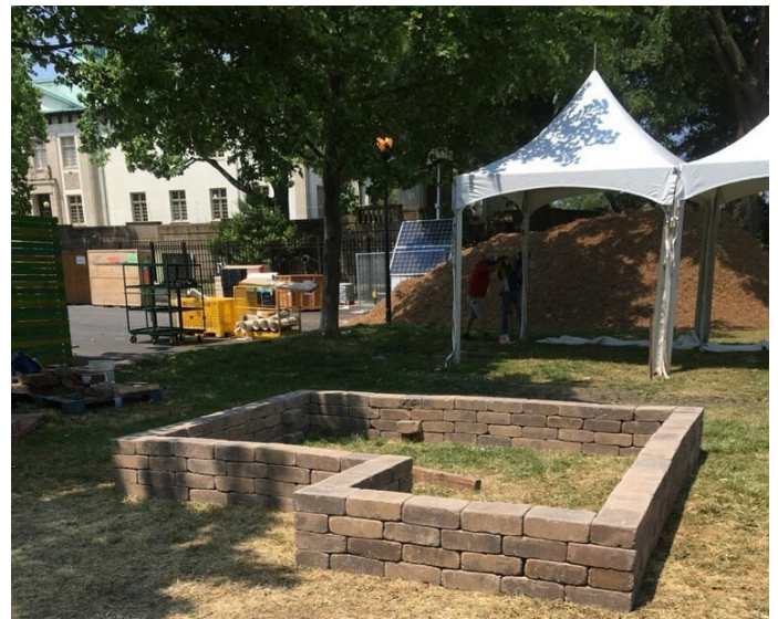
Walls are done!
